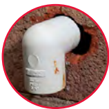
Structural repair (exclusion)
